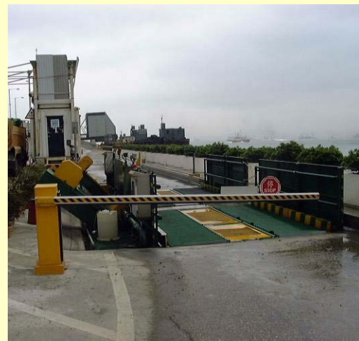
DWA-05 起落閘 Auto Gate Barrier
